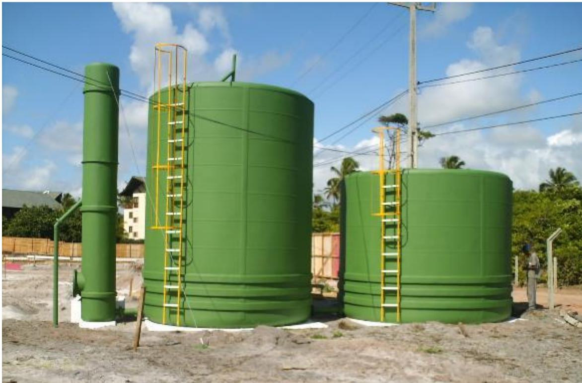
Figura 14 - Reator UASB
